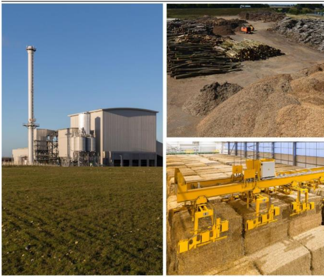
Picture credit: left and lower right: Snetterton biomass power plant, UK, by courtesy of Burmeister & Wain Scandinavian Contractor A/S, upper right: biomass storage area at the biomass power plant Nesle- Douard, by courtesy of CNIM Waste & Energy Management Solutions (WEMS).
